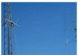
One half of the new 75/80-meter cage antenna going up at W1AW. The antenna is suspended on three of W1AW's towers.
